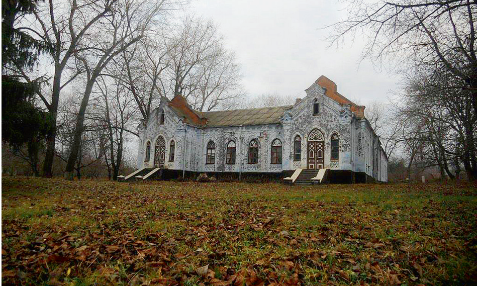
Photo 4. The parish school building of Kazimir mansion from Cernoleuca village in Dondușeni district Source: Tarhon, 2013
